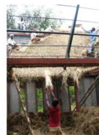
Fig.7: Thatching of roof. Source: Pragrup
