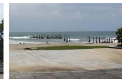
Fig 09: Dilapidated piers, Source: Amrutha, 2021
