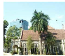
Fig. 4. The stone church in contrast to glass and steel Source : Google photos
