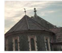
Fig. 9. Panorama of roof with arch windows Source : Google photos
