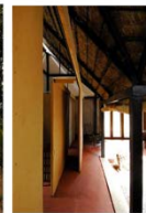
Fig.9: Re-engineered wooden partitions. Source: Pragrup
