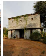
Fig.8: Front façade. Source: Pragrup
