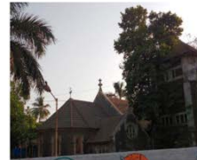
Fig. 8. Panorama of timber roof with mangalore tiles Source : Google photos
